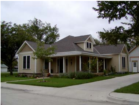
New infill residential construction
