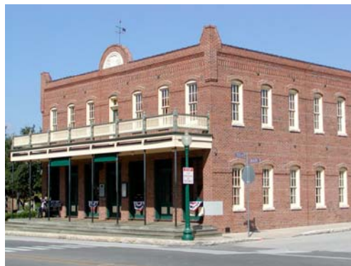
Reconstruction of a historic building
